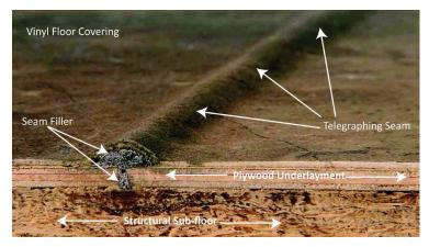
Fastener blow-through is caused by not properly adjusting the drive depth or air pressure in your staple or nail gun which can result in shooting the fastener completely through the underlayment. Nothing short of physical plywood failure such as a delamination will be warranted with regard to telegraphing seams.
